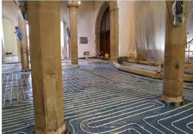
The work to install the under floor heating system took place over four months in 2011. The church was closed for the contract period. The pews were removed and the floor lifted. The 'floor' was then dug down to a depth of about three feet; a layer of hardcore was laid on which was put a layer of concrete. A layer of insulation was put upon the concrete, then the plastic heating pipes were coiled and more concrete was laid on top. It was finally finished with a York stone floor.
